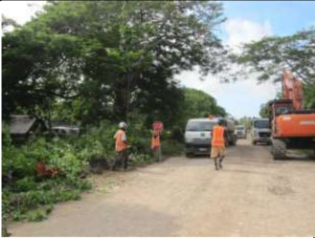
Clearing vegetation from the new road corridor in Eton Village.
