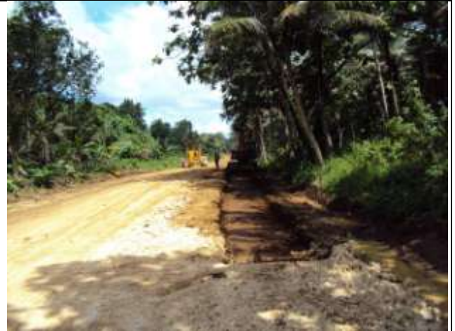
Santo: Widening the road near the 40 km mark.
