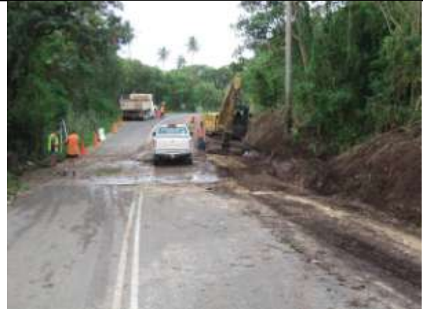
Efate: Lakenasua Floodway. Excavating the upstream side of the reconstructed structure.
