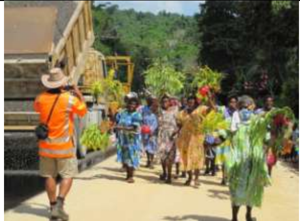
Progress with sealing on Santo – here Hog Harbour mamas celebrate the sealing of the road through their village.
