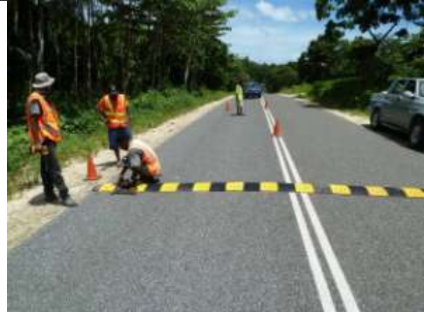
Installing a speed bump in Hog Harbour.
