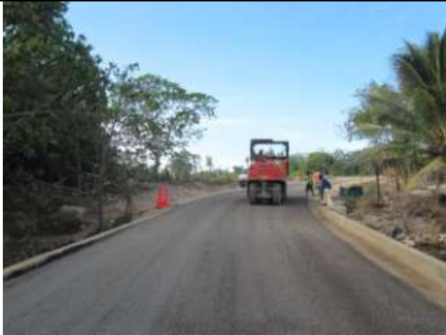
Sealing progress: The seal operation reaches the bridge at Sara Beach. Sealing will continue to the Epule area.
