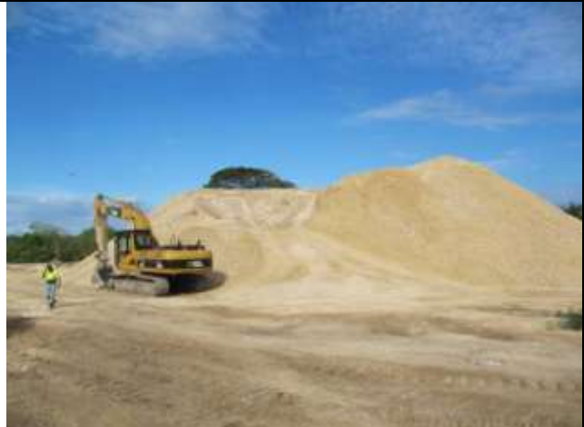
Quarry Foreman Jack Sharon (left foreground) is dwarfed by the 17,000 m 3 coral aggregate stockpile at Epule. This will sustain the pavement work while the quarry plant relocates to the next site.
