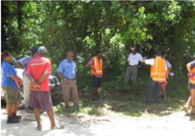
MCA and Downer staff discuss the Santo East Coast road works in the Hog Harbour area, following good feedback from the local community.
