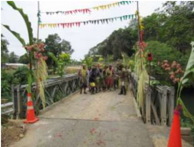
Epule and Matarisu custom dancers assembling on the decorated Epule Bailey Bridge to celebrate progress with the sealing of the road.
