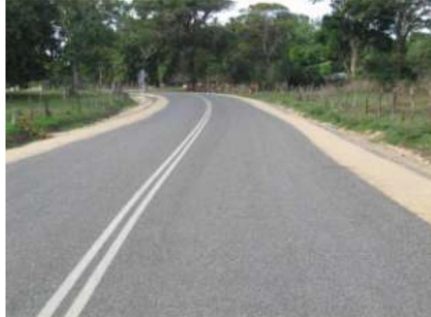
Double solid line. This means it is **NOT** safe to overtake in any direction. Photo taken near Epule.
