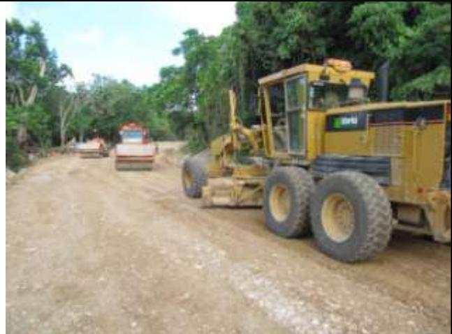
Shaping and compacting the pavement near the 58 km mark between Epau and Pangpang.
