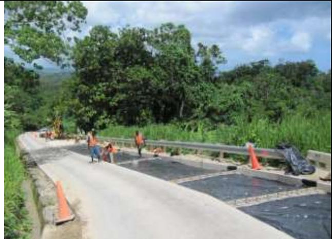
Klehm's Hill – just below the corner halfway up the hill – preparing the pavement panels for pouring. This work is now 75 % complete.
