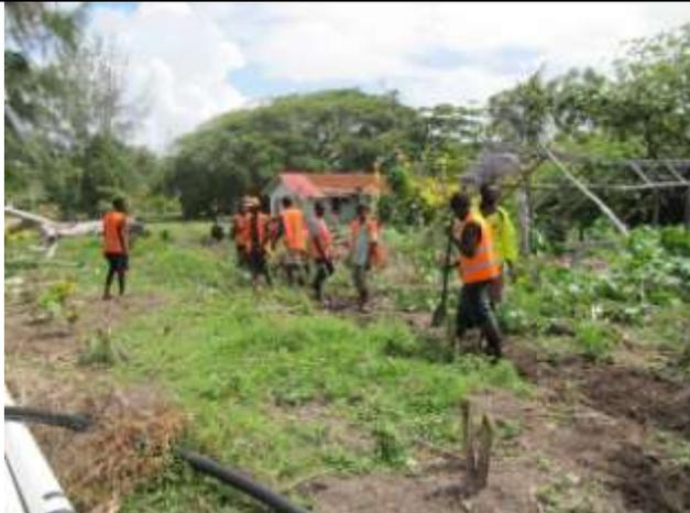
The Eton village water pipe crew. There are a number of water pipes alongside the road through the village that will be affected by the road widening. This team is relocating the water pipes so that they are clear of the roadway in advance of construction work reaching the village.
