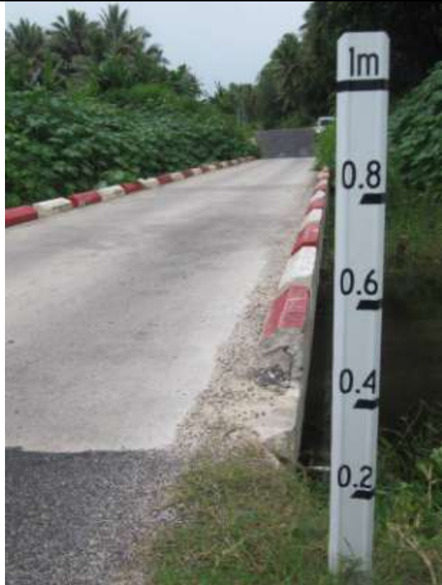
Flood Depth Indicator. The figures show the depth in meters that the flood water is above the normal road surface. Caution and judgment are required whenever driving through flood waters. If in doubt wait for the flood to pass.
