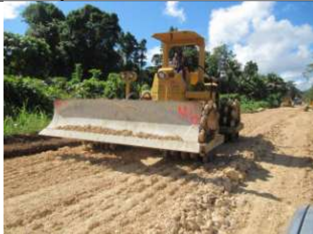
Santo: Compacting and shaping pavement near the 39 km mark, South of Hog Harbour.
