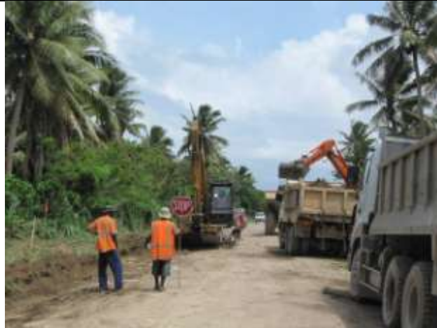
Efate: Clearing underway at Nangus – just South of Eton Village.
