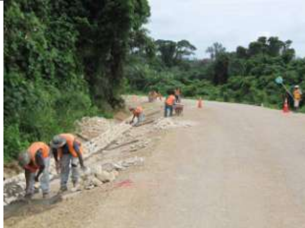
Efate: Rock lined drain construction underway near Forari.
