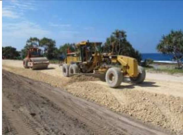
A Downer grader (operated by Johnathan How) and roller (operated by Edward Tasaruru) shaping & compacting pavement near Dry Creek in East Efate
