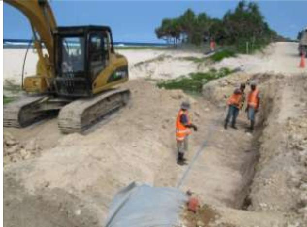
Preparing to install gabions at Dry Creek, from left to right, Rose David, “Pin” Chandra and Wesley Timas check the dimensions of the excavation. In the background Joshua Matai makes up the wire gabion baskets.
