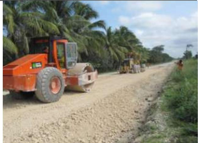
Downer roller and grader compacting and shaping pavement at Banana Bay. On the right Abel Reynolds uses a level to check the pavement as it is laid.
