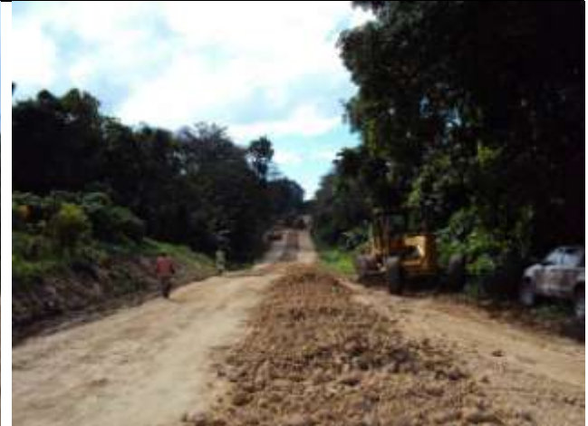
Santo. Overlaying the widened pavement just North of Hog Harbour village.
