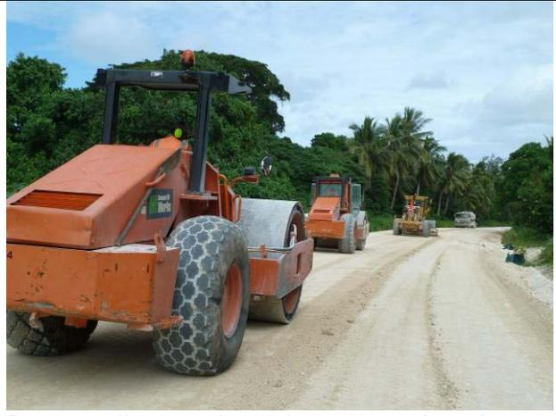
Downer rollers, grader and a water truck work on the final section of unsealed pavement near Eton Beach.
