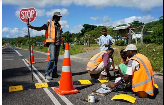
Installing speed bumps in Tanoliu. These are a trial to see how the bumps perform, especially to determine how effective they are at slowing traffic down.
