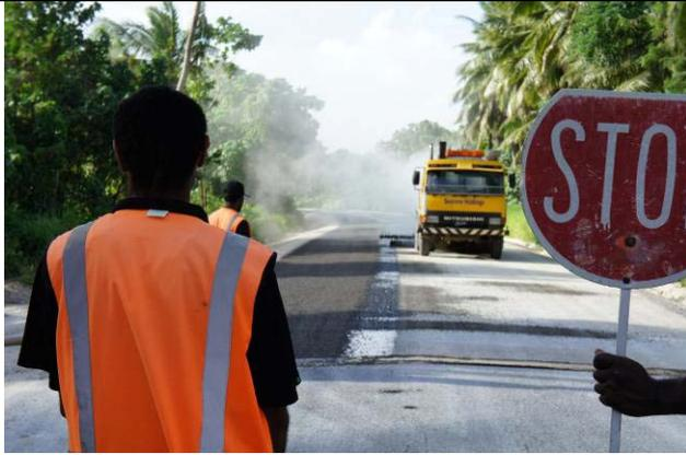
Applying the first seal coat near Nangus (close to Eton Village).
