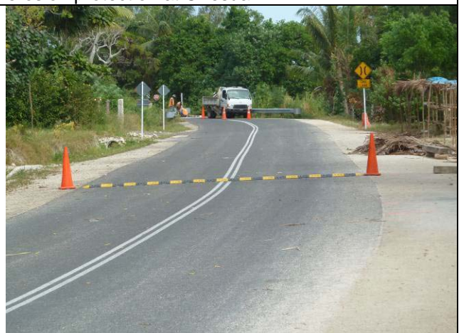
Speed bumps made of plastic, instead of the conventional concrete are being trialled at Tanoliu.
