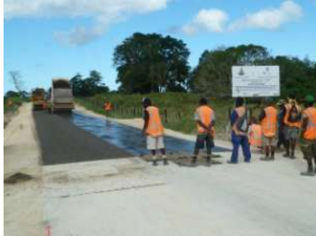
Spreading black stones on the freshly sprayed bitumen.
