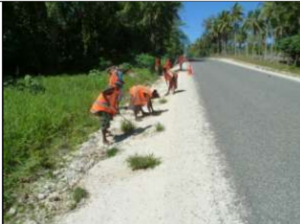
Transplanting grass into the table drain to encourage vegetation to grow near the Blue Lagoon. This work is being done by a crew of girls from Eton Village.
