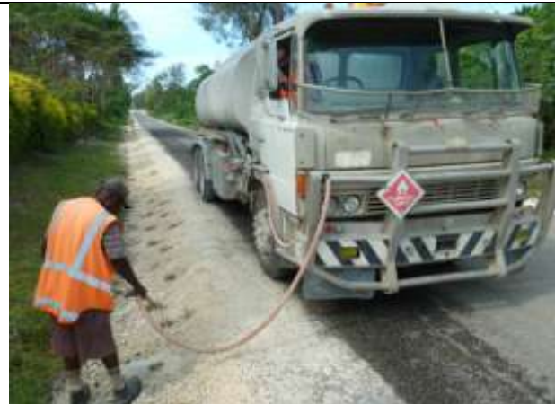
Joseph Noviel and Obed Ben water the newly transplanted grass in the table drains near Eton.
