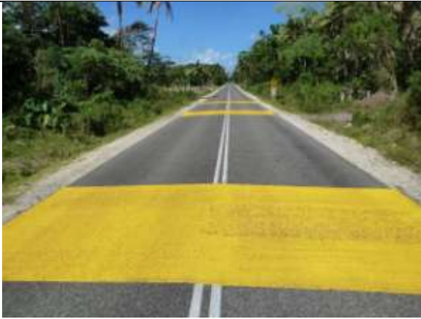
Speed calming at Paonangisu - the bright markings and large sized sealing chip are intended to warn motorists of the many pedestrians and 30 km/hr speed limit in the section between Manua School and the Paonangisu Health Centre.
